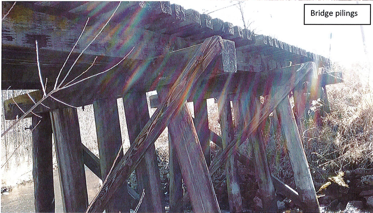
Bridge from SW edge of abutment
